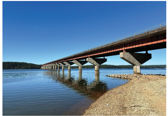
Fig. 1: John Coffee Memorial Bridge
