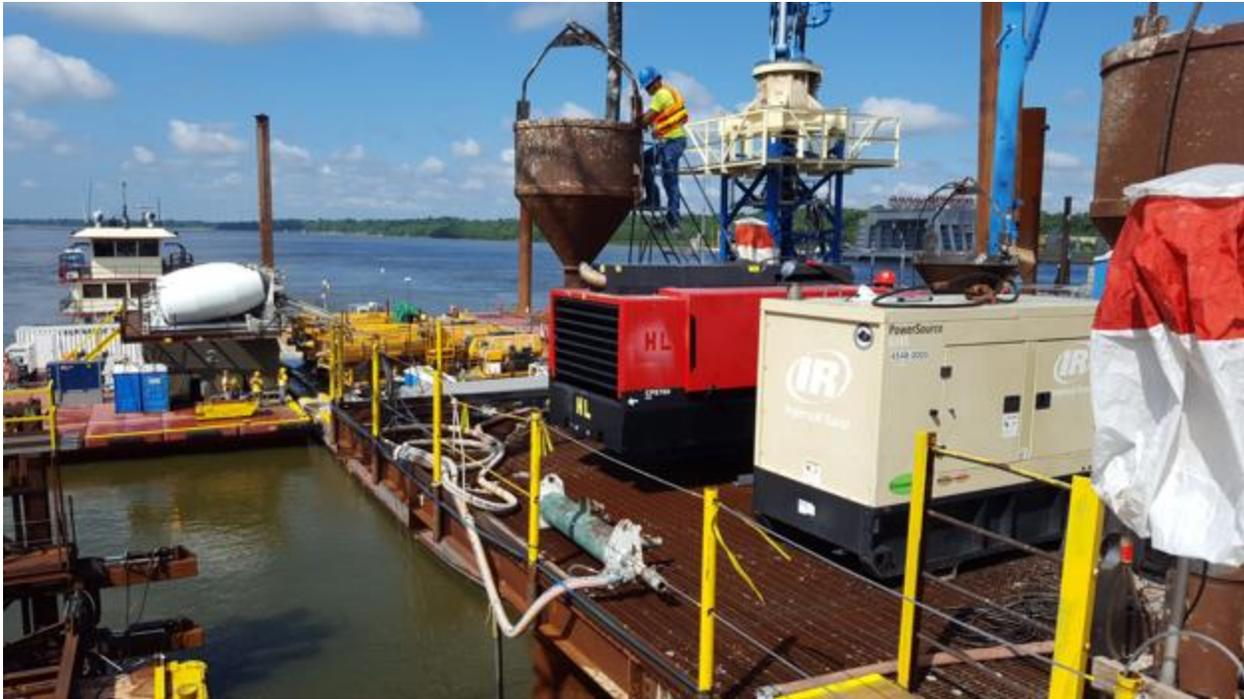
**Figure 3**—Tremie Concrete Placement at Olmstead Dam in August 2016 (Source: U.S. Army Corps of Engineers)
