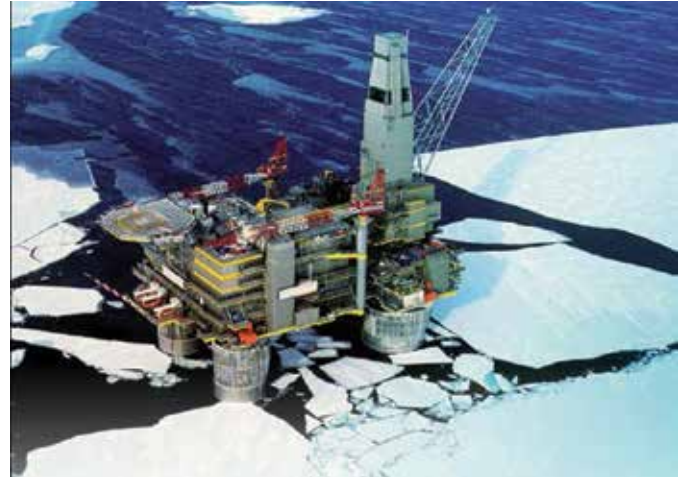
Fig. 4: Sea ice impacts the Sakhalin II LUN-A Platform, Russia (photo courtesy of Kvaerner)
